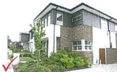
Example of compliant treatment, articulation of corner and verandah wrapping the corner.
