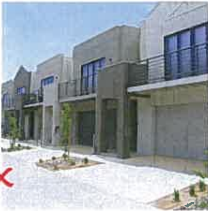
Example of non compliant treatment, no setbacks.
