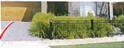
Example of compliant front fencing, greater than 50% transparent and less than 1.2m in height.
