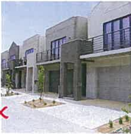
Example of non compliant treatment, no setback.
