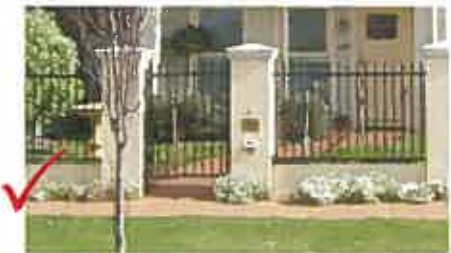
Example of compliant letterbox.
