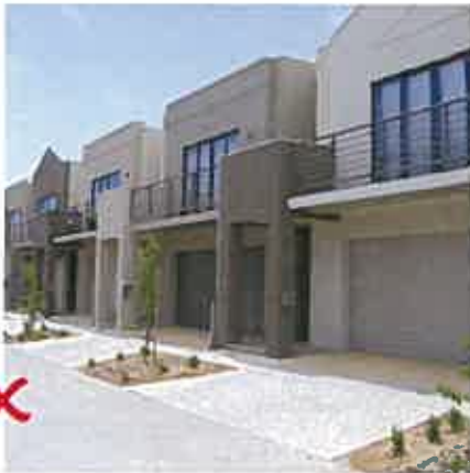
Example of non compliant treatment, no setback.
