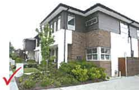
Example of compliant treatment, articulation of corner and verandah wrapping the corner.
