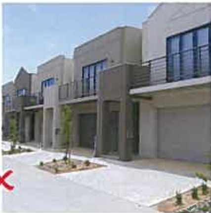
Example of non compliant treatment, no setback.
