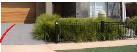
Example of compliant front fencing, greater than 50% transparent and less than 1.2m in height.
