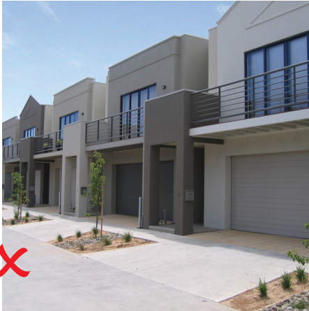
Example of non compliant treatment, no setback.
