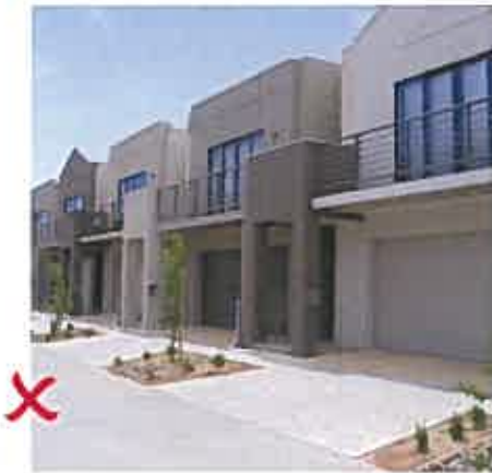
Example of non compliant treatment, no setback.
