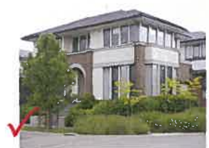
Example of compliant treatment, articulation of corner and verandah wrapping the corner.
