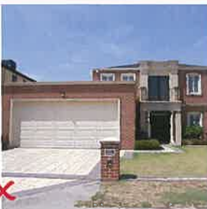
Example of non compliant treatment for garage, set forward from the main built form.
