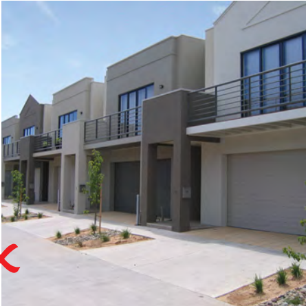
Example of non compliant treatment, no setback.
