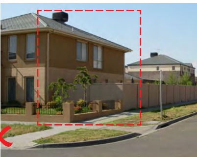
Example of non compliant treatment, no articulation or addressing open space.
