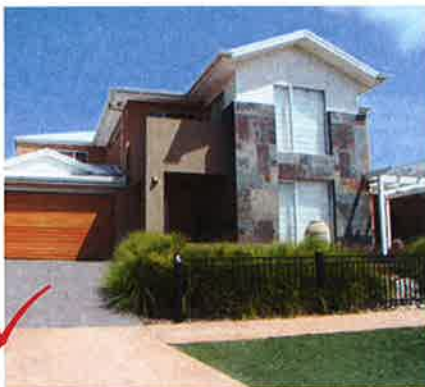
Example of compliant front fencing, greater than 50% transparent and less than 1.2m in height.
