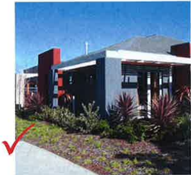
Example of compliant treatment, articulation of corner and verandah wrapping the corner.
