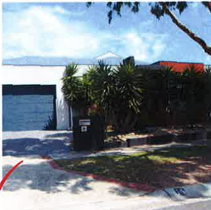
Example of compliant letterbox.
