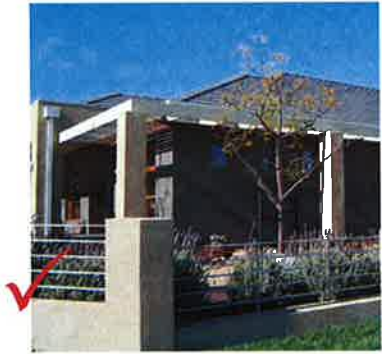
Example of compliant treatment, articulation of corner and verandah wrapping the corner.
