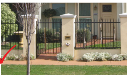
Example of compliant letterbox.
