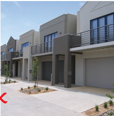
Example of non compliant treatment, no setback.
