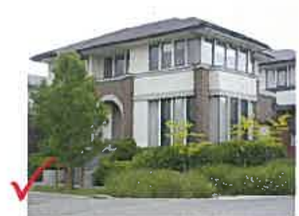
Example of compliant treatment, articulation of corner and verandah wrapping the corner.
