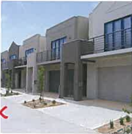
Example of non compliant treatment, no setback.
