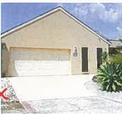
Example of non-compliant treatment for porches and entries, no features.
