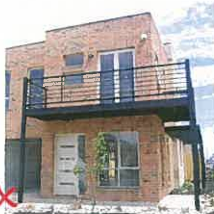
Example of non-compliant material treatment, no differentiation materials.
