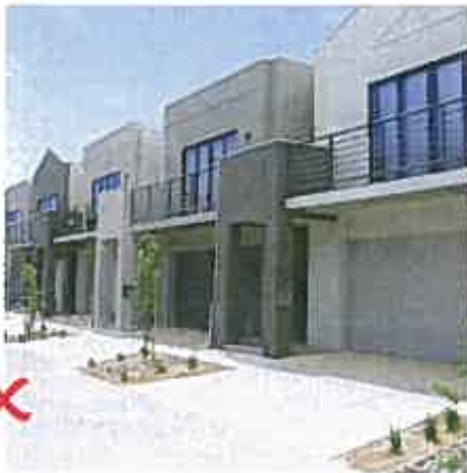
Example of non compliant treatment, no setbacks.
