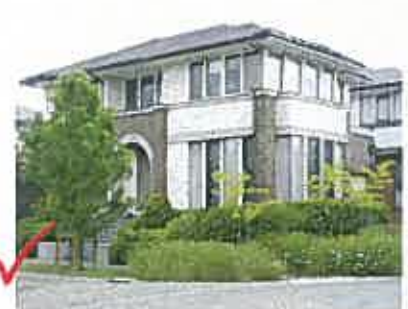
Example of compliant treatment, articulation of corner and verandah wrapping the corner.
