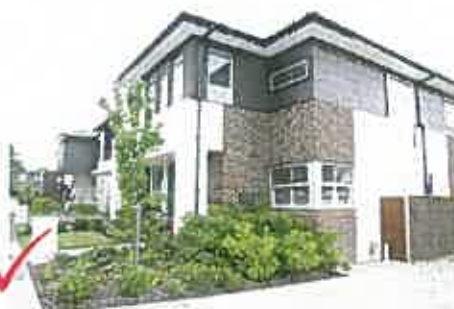
Example of compliant treatment, articulation of corner and verandah wrapping the corner.
