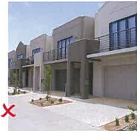
Example of non compliant treatment, no setback.
