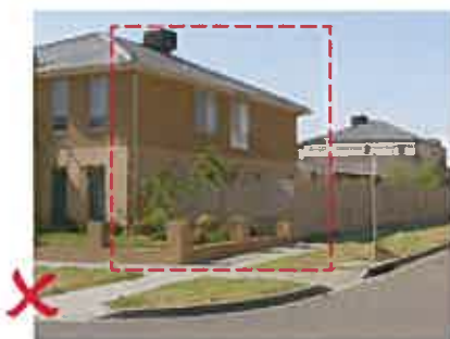
Example of non compliant treatment, no articulation or addressing open space.
