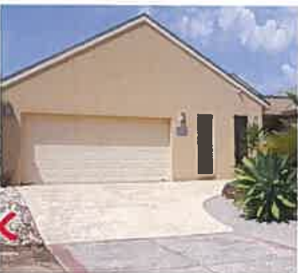
Example of non-compliant treatment for porches and entries, no features.
