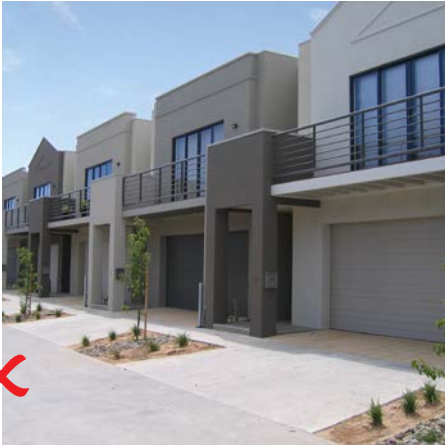
Example of non compliant treatment, no setback.
