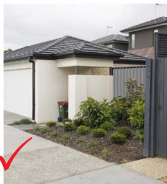
Example of compliant treatment for rear lane (metal fencing and gate access).
