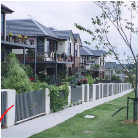
Example of compliant treatment for small lot setbacks, overlooking open space.
