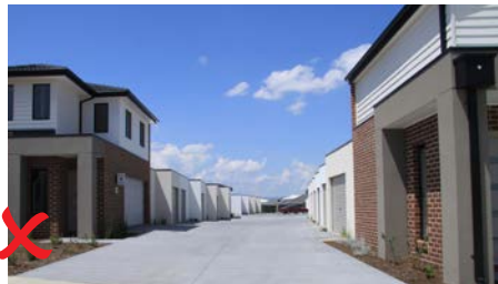
Example of non-compliant treatment for rear lane.
