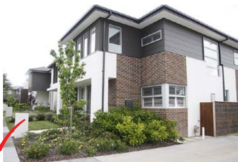
Example of compliant treatment, articulation of corner and verandah wrapping the corner.
