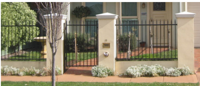
✓ Example of compliant letterbox.
