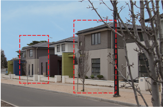
X Example of non compliance façades, identical façades to close together
