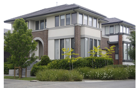
✓ Example of compliant treatment, articulation of corner and verandah wrapping the corner.
