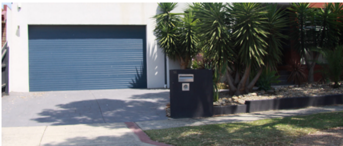
✓ Example of compliant letterbox.
