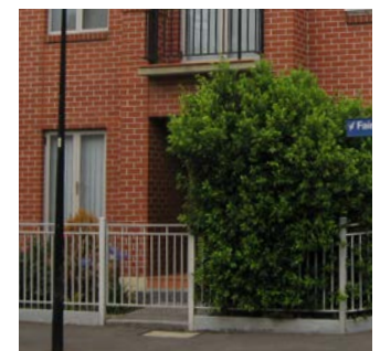
Example of front fence not in accordance with these guidelines
