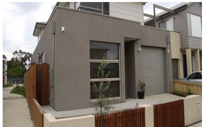
Example of meter box colour and hot water tank location in accordance with these guidelines
