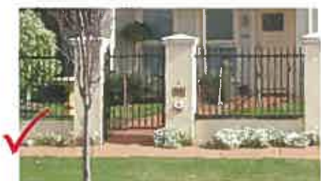
Example of compliant letterbox.
