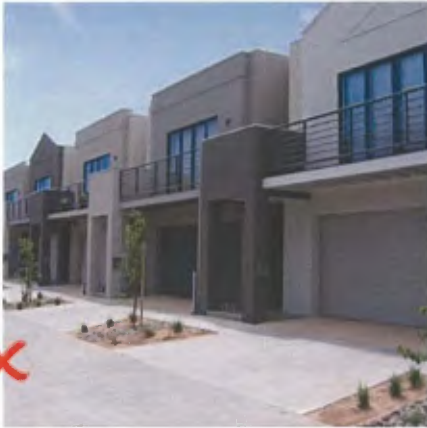
Example of non compliant treatment, no setback.
