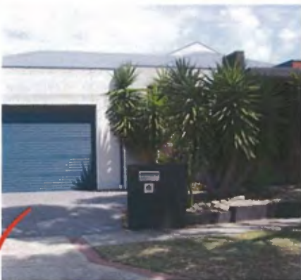
Example of compliant letterbox.
