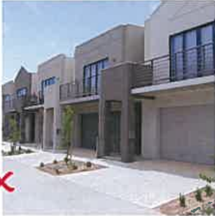
Example of non compliant treatment, no setback.
