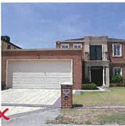
Example of non compliant treatment for garage, set forward from the main built form.
