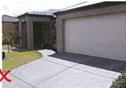
Example of non compliant driveway, plain concrete not permitted.
