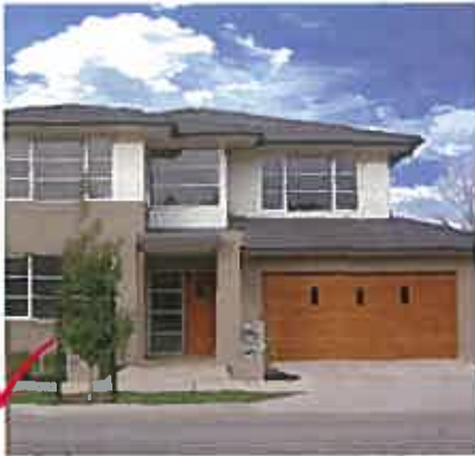
Example of compliant treatment for garage, integrated into, and complements built form character.
