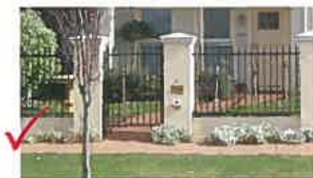
Example of compliant letterbox.
