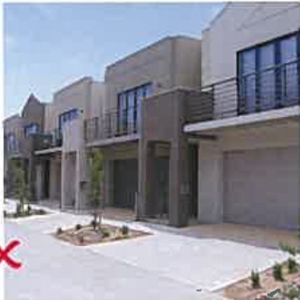
Example of non compliant treatment, no setback.
