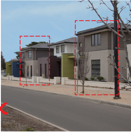
Example of non compliance facades, identical facades to close together
