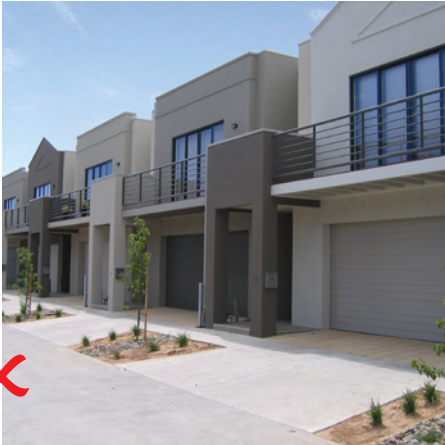
Example of non compliant treatment, no setback.
