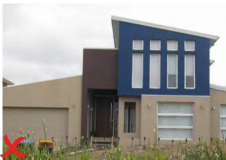
Example of non compliant colour scheme
