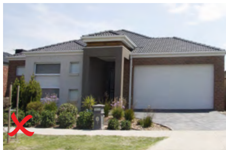
Example of non compliant treatment no eaves
