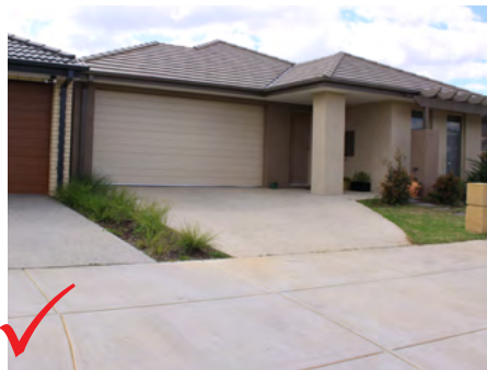
Example of compliant treatment for garage, slimline door
