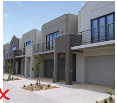
Example of non compliant treatment, no setback.
