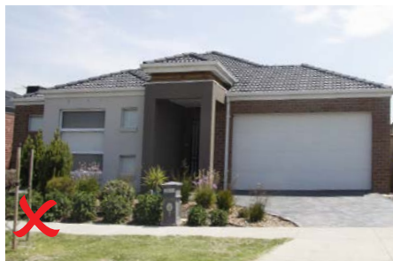
Example of non compliant treatment no eaves
