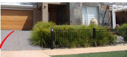
Example of compliant front fencing, greater than 50% transparent and less than 1.2m in height.
