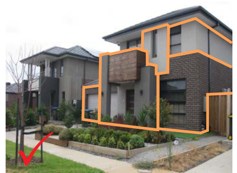
Articulated building forms
