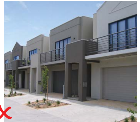
Example of non compliant treatment, no setback.
