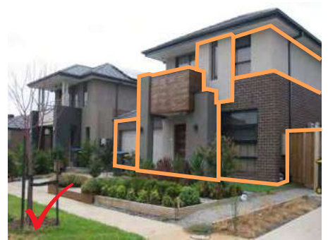
Articulated building forms
