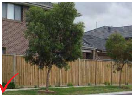
Example of compliant timber paling fence with capping, exposed posts and palings fronting the street
