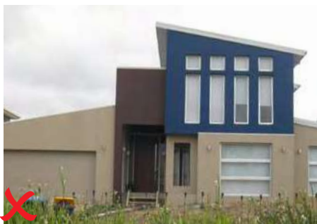
Example of non compliant colour scheme
