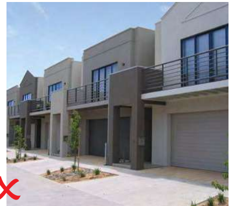
Example of non compliant treatment, no setback.
