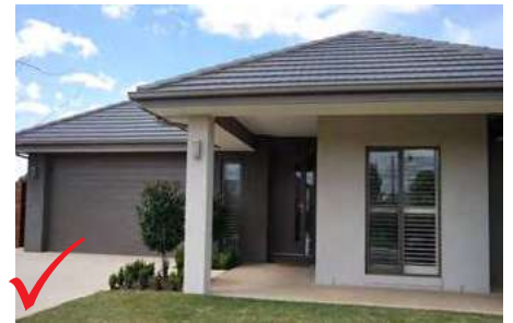
Example of eaves that overhang the dwelling facades that face the street
