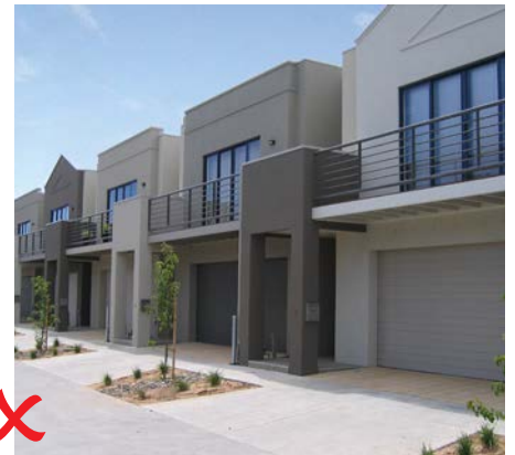
Example of non compliant treatment, no setback.
