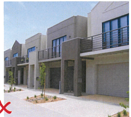
Example of non compliant treatment, no setback.
