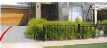
Example of compliant front fencing, greater than 50% transparent and less than 1.2m in height.
