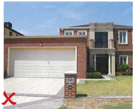
Example of non compliant treatment for garage, set forward from the main built form.
