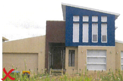
Example of non compliant colour scheme
