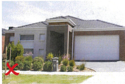
Example of non compliant treatment no eaves
