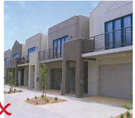
Example of non compliant treatment, no setback.
