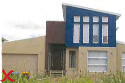
Example of non compliant colour scheme
