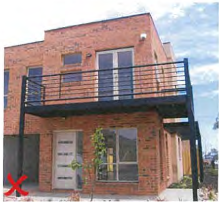
Example of non compliant materials treatment, no differentiating materials.
