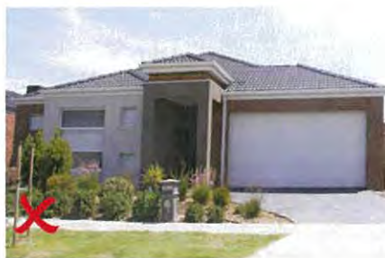
Example of non compliant treatment no eaves
