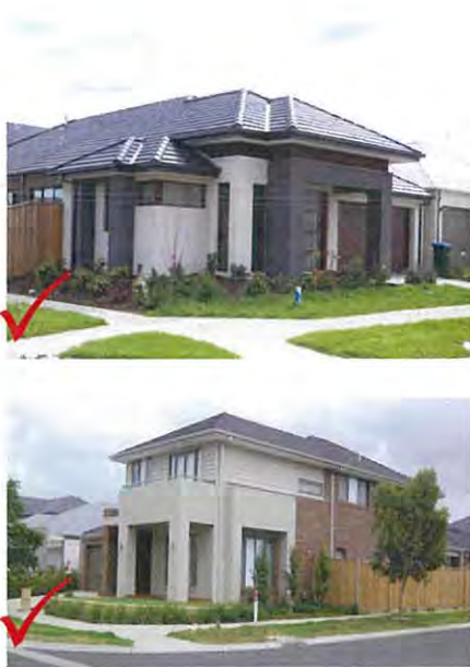
Examples of single and double storey houses on corner lots that address both street frontages with well-articulated architectural elements, such as the verandahs and windows. Double storey dwellings also utilise a variation of building material on both facades breaking down the scale of the building.
