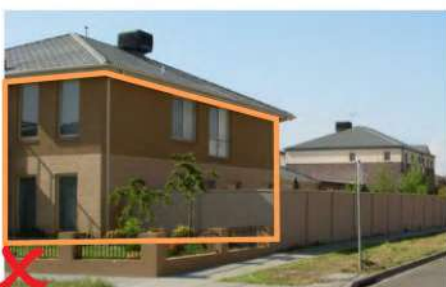
Example of non compliant treatment, no articulation or addressing open space.
