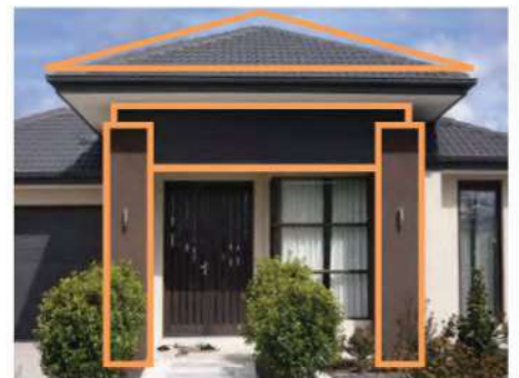
Facade detailing with contemporary awnings
