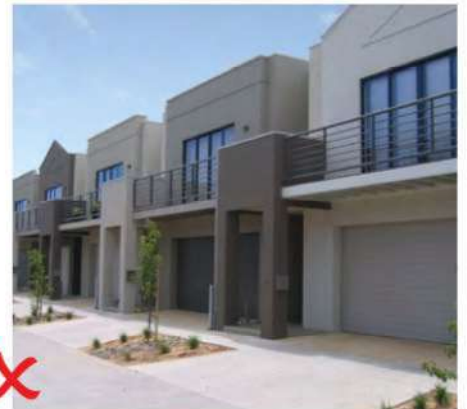
Example of non compliant treatment, no setback.
