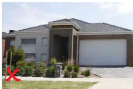
Example of non compliant treatment no eaves
