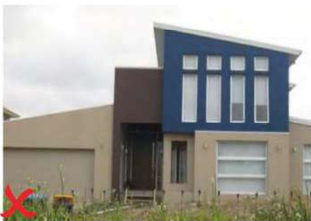
Example of non compliant colour scheme
