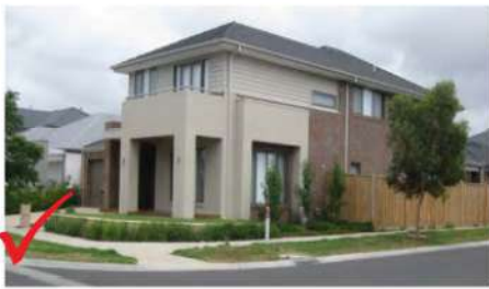
Examples of single and double storey houses on corner lots that address both street frontages with well-articulated architectural elements, such as the verandahs and windows. Double storey dwellings also utilise a variation of building material on both facades breaking down the scale of the building.
