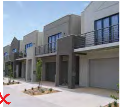
Example of non compliant treatment, no setback.
