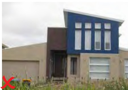
Example of non compliant colour scheme
