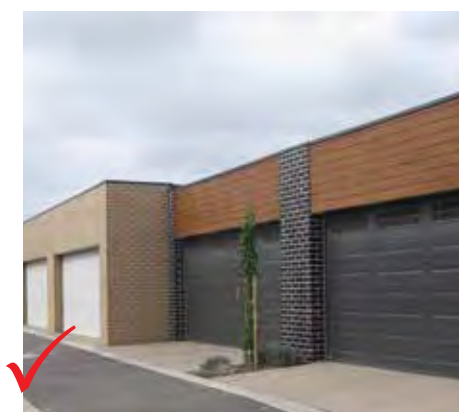
Example of compliant garage setback.
