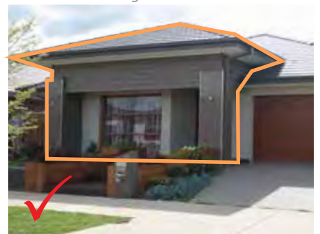
Facade detailing with contemporary awnings
