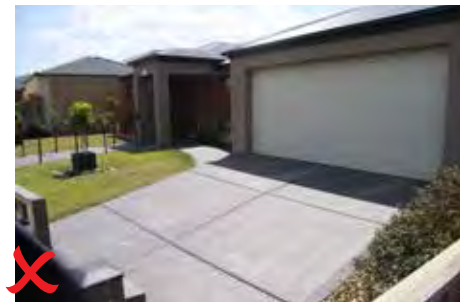
Example of non compliant driveway, plain concrete not permitted.
