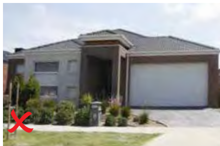
Example of non compliant treatment no eaves
