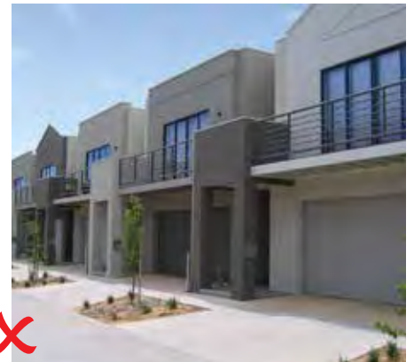
Example of non compliant treatment, no setback.
