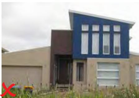
Example of non compliant colour scheme
