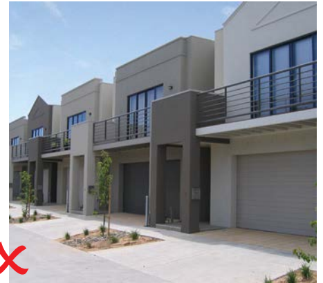
Example of non compliant treatment, no setback.
