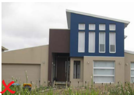
Example of non-compliant colour scheme
