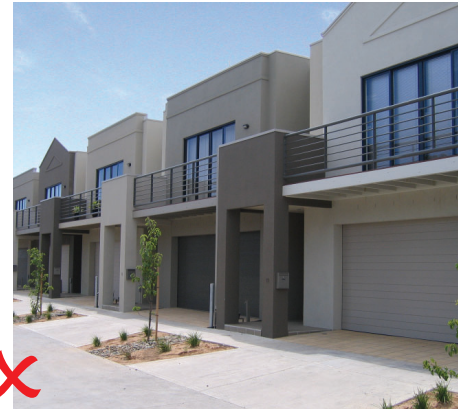
Example of non compliant treatment, no setback.
