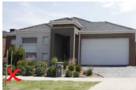
Example of non compliant treatment no eaves
