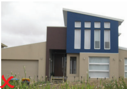
Example of non-compliant colour scheme
