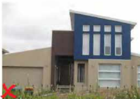
Example of non-compliant colour scheme
