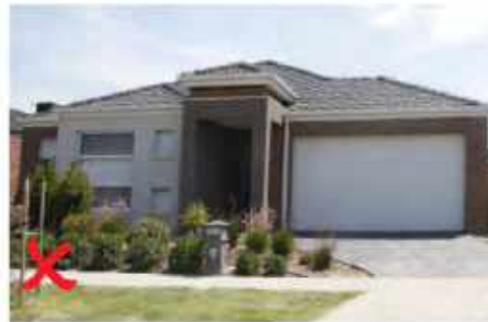
Example of non compliant treatment no eaves
