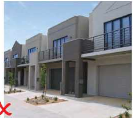
Example of non compliant treatment, no setback.
