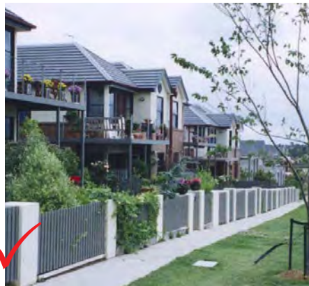
Example of compliant treatment for small lot setbacks, overlooking open space.
