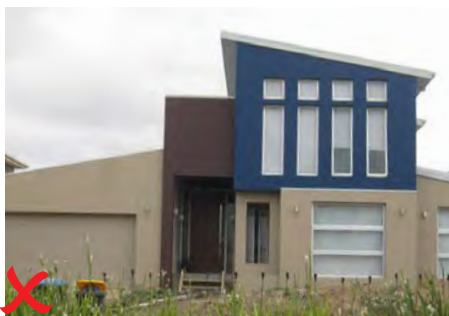
Example of non-compliant colour scheme
