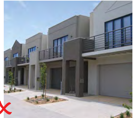
Example of non compliant treatment, no setback.
