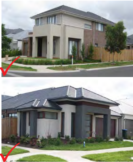
Examples of single and double storey houses on corner lots that address both street frontages with well-articulated architectural elements, such as the verandahs and windows. Double-storey dwellings also utilise a variation of building material on both facades breaking down the scale of the building.
