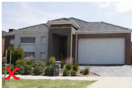
Example of non compliant treatment no eaves
