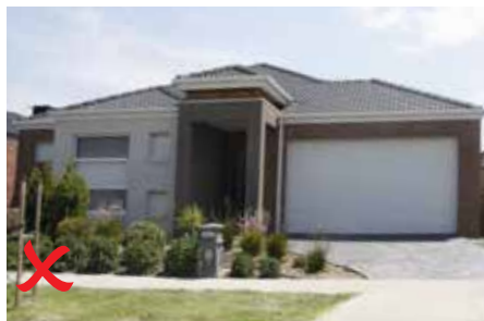
Example of non compliant treatment no eaves
