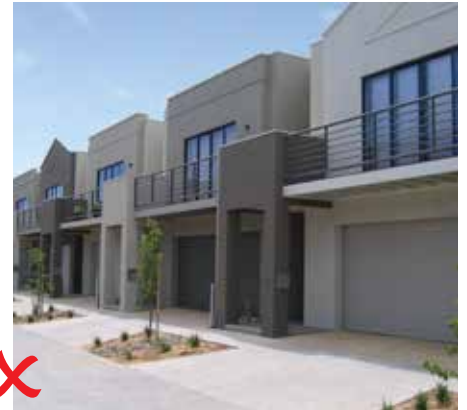
Example of non compliant treatment, no setback.
