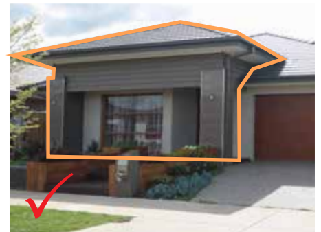
Facade detailing with contemporary awnings
