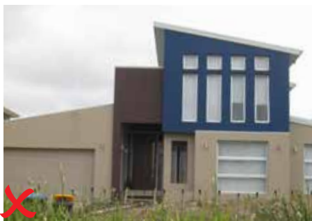
Example of non-compliant colour scheme
