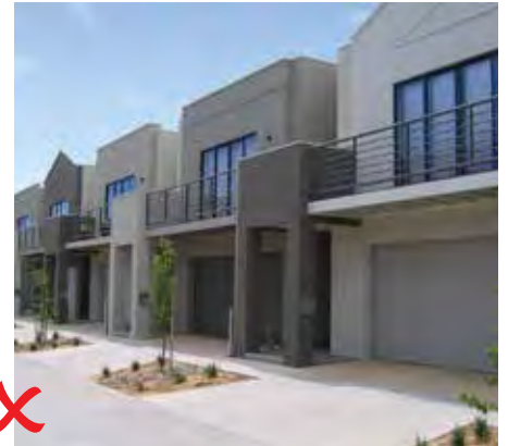
Example of non compliant treatment, no setback.
