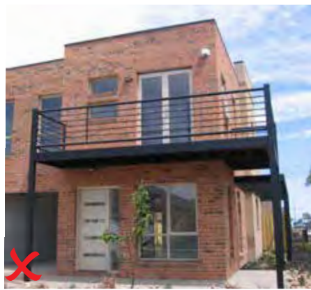
Example of non compliant materials treatment, no differentiating materials.
