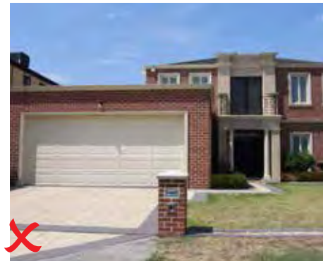
Example of non compliant treatment for garage, set forward from the main built form.
