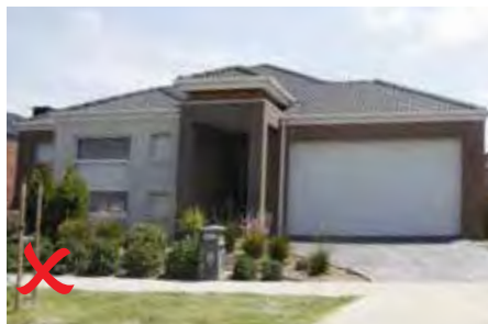
Example of non compliant treatment no eaves
