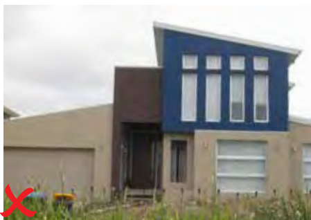
Example of non-compliant colour scheme
