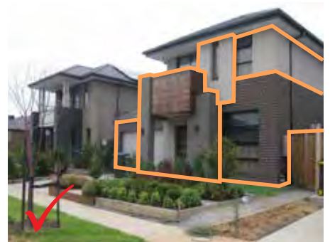
Articulated building forms
