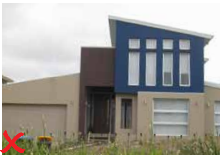
Example of non-compliant colour scheme
