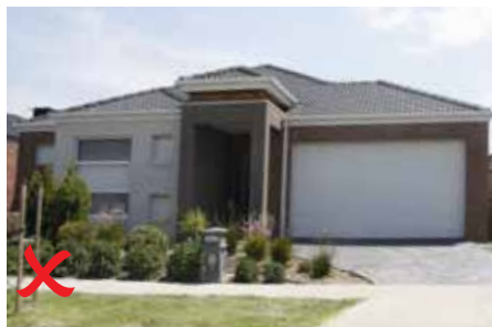
Example of non compliant treatment no eaves
