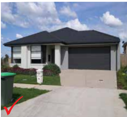
Garage setback from street frontages and behind front wall of the home.
