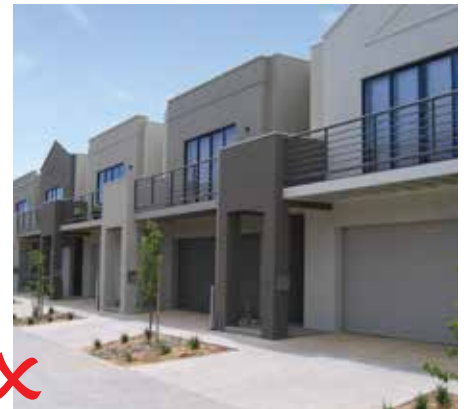
Example of non compliant treatment, no setback.
