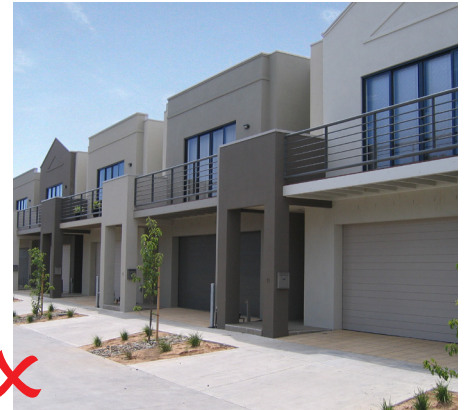
Example of non compliant treatment, no setback.
