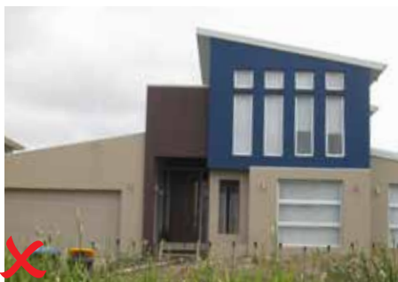
Example of non-compliant colour scheme
