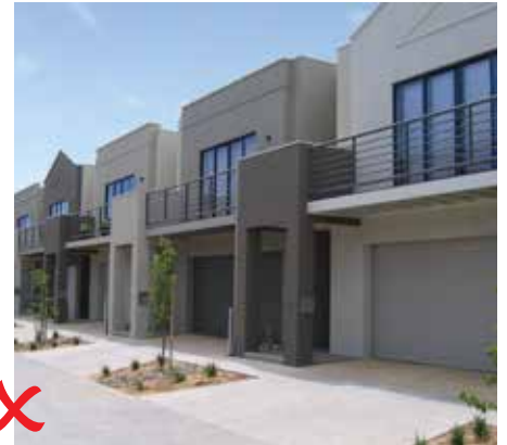
Example of non compliant treatment, no setback.
