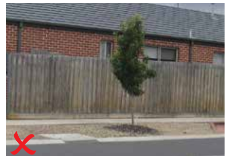
Example of non compliant timber paling fence without capping and exposed posts
