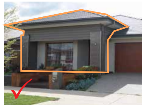
Facade detailing with contemporary awnings
