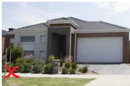
Example of non compliant treatment no eaves
