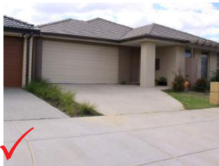
Example of compliant treatment for garage with slimline door.
