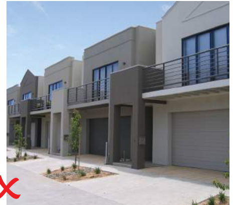
Example of non compliant treatment, no setback.
