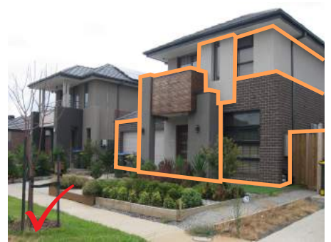
Articulated building forms
