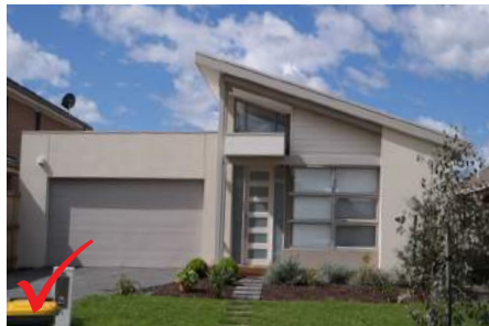
Example of skillion roof
