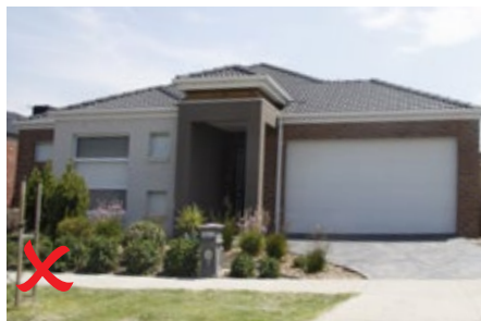
Example of non compliant treatment no eaves
