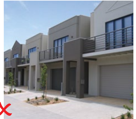
Example of non compliant treatment, no setback.
