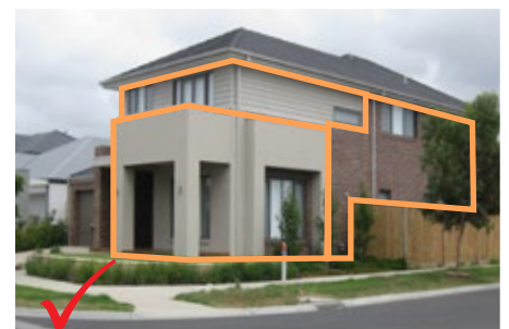
Complementary building materials
