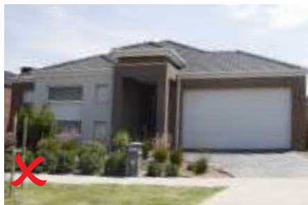
Example of non compliant treatment no eaves
