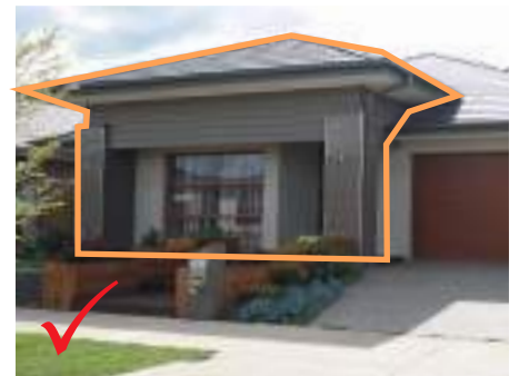
Facade detailing with contemporary awnings
