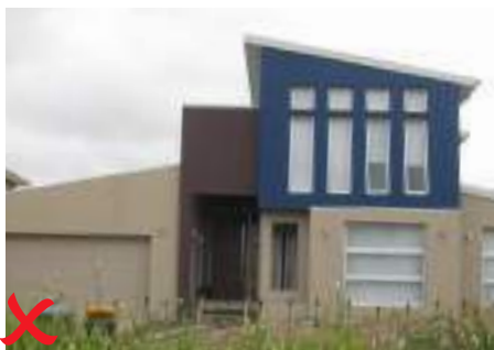
Example of non-compliant colour scheme
