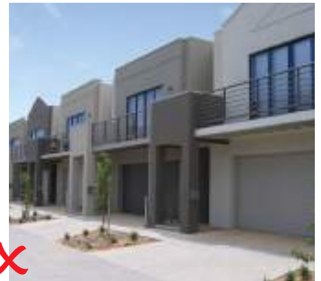
Example of non compliant treatment, no setback.
