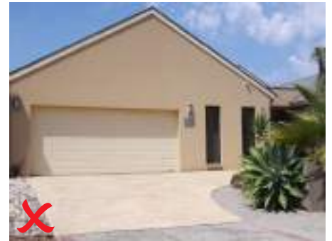
Example of non compliant treatment for porches and entries, no features.
