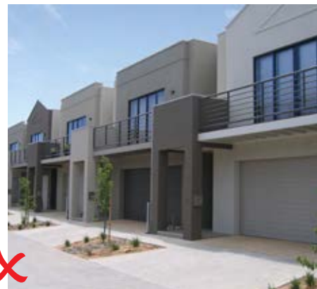
Example of non compliant treatment, no setback.
