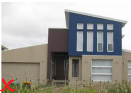
Example of non-compliant colour scheme
