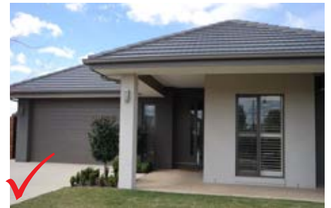
Example of eaves that overhang the dwelling facades that face the street
