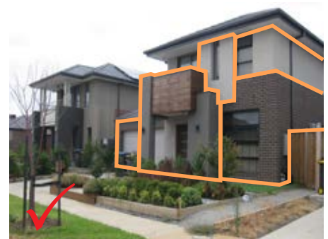
Articulated building forms
