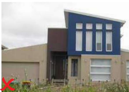
Example of non-compliant colour scheme
