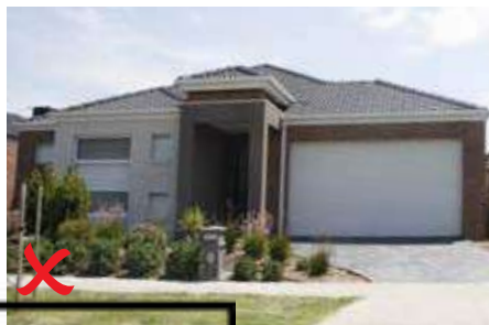
Example of non compliant treatment no eaves
