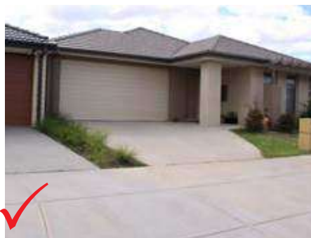
Example of compliant treatment for garage with slimline door.
