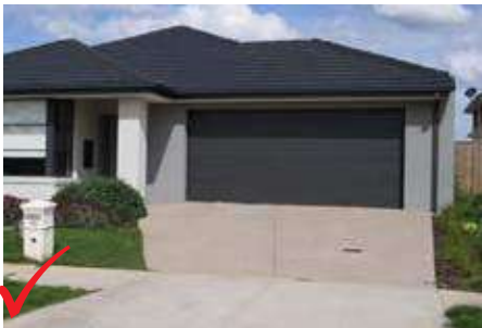
Example of compliant driveway, tapered to align with the crossover.
