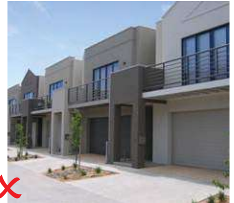
Example of non compliant treatment, no setback.
