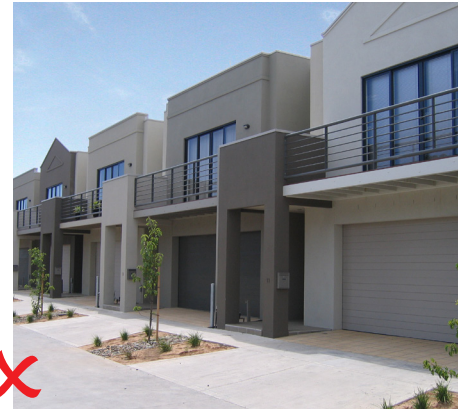
Example of non compliant treatment, no setback.
