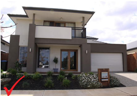
Double storey dwelling with garage incorporating 1.5m covered verandah/ balcony, hence not requiring setback between the front wall and garage.
