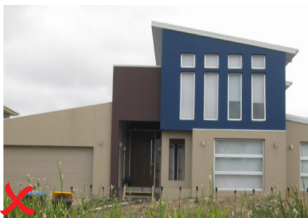
Example of non-compliant colour scheme
