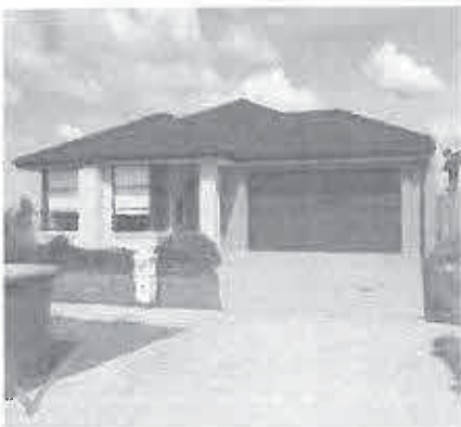
Garage setback from street frontage, and behind front wall of the house.
