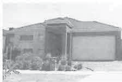
Example of non compliant treatment: no eaves
