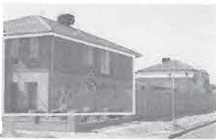
Example of non compliant treatment, no articulation of address to open space.
