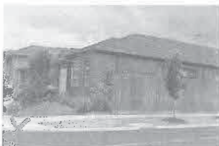
Example of non-compliant standard lot corner treatment.
