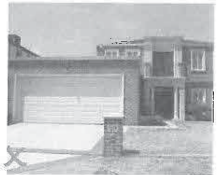
Example of non compliant treatment for garage, set forward from the main built form.
