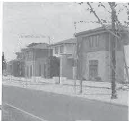
Example of non compliance façades, identical façades too close together
