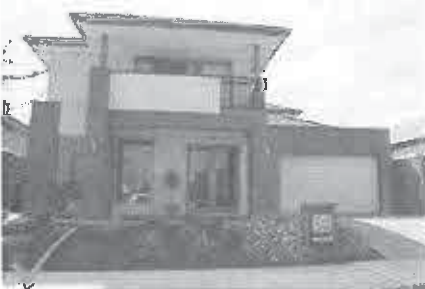
Double storey dwelling with garage incorporating 1.5m covered verandah/ balcony, hence not requiring setback between the front wall and garage.
