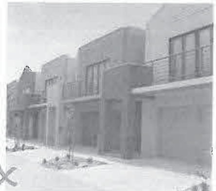
Example of non compliant treatment, no setback.
