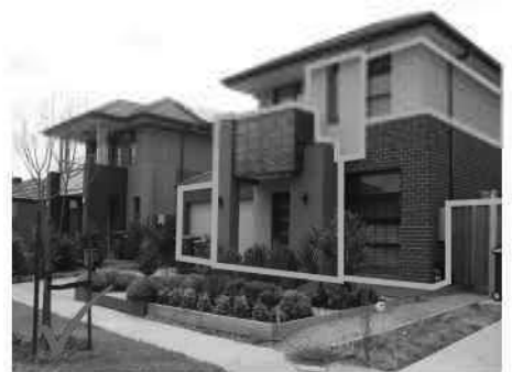
Articulated building forms
