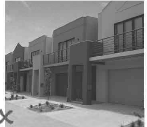
Example of non compliant treatment, no setback.
