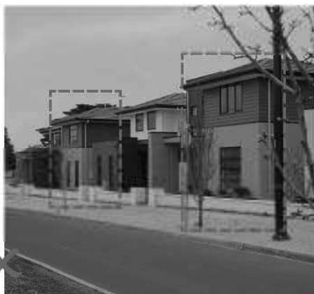
Example of non compliance facades, identical facades too close together
