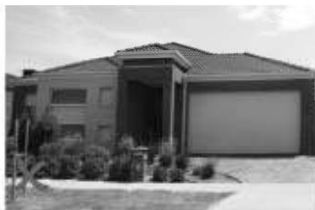
Example of non compliant treatment no eaves
