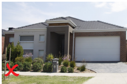
Example of non compliant treatment no eaves
