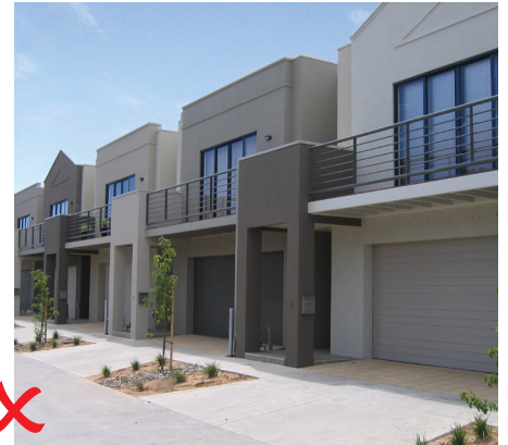
Example of non compliant treatment, no setback.
