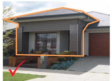
Facade detailing with contemporary awnings
