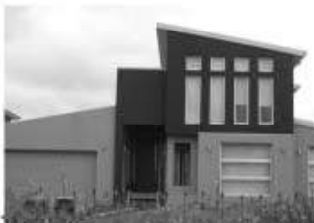
Example of non-compliant colour scheme
