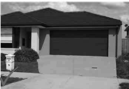
Example of compliant driveway, tapered to align with the crossover.
